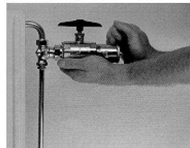
3. While continuing to press in on the stem handle, engage the thread of the union tailpiece of the changer with the thread on the neck of the valve. Turn the changer onto the valve neck until it is firmly in place and sealed.
