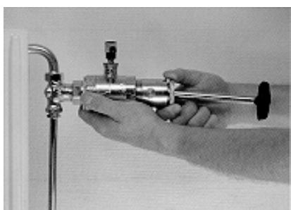
7. Holding the changer so that it does not turn, turn the bonnet out of the chamber.
